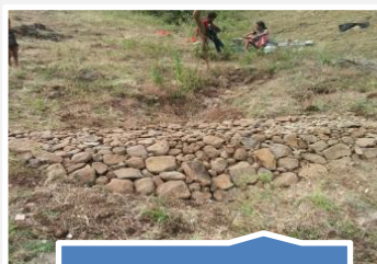
GULLY PLUG WORK
